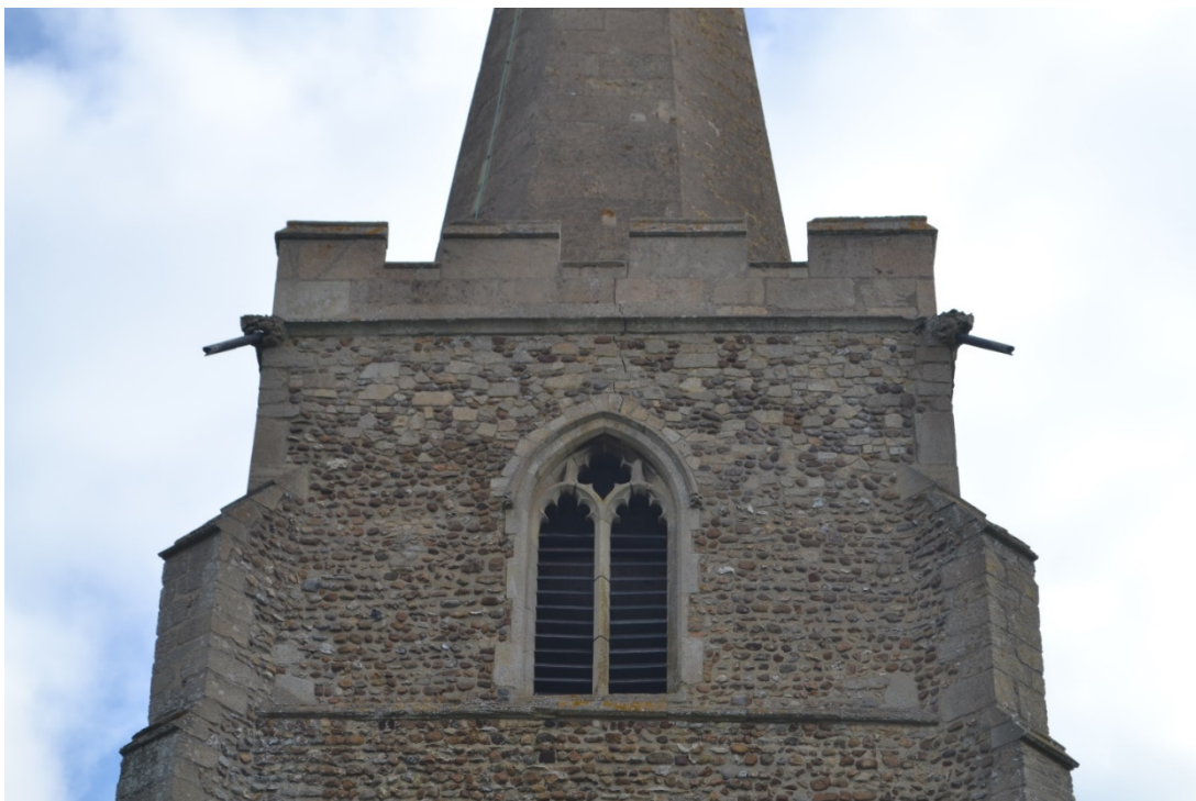
Photograph 6.7: All Saints Church. Cracks above the church window are visible in this photograph
