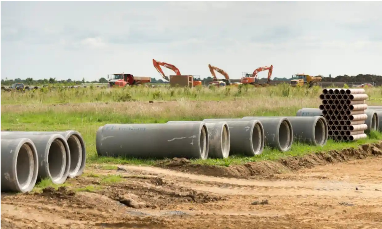
Construction work at Northstowe, north-west of Cambridge. Photograph: Julian Eales/Alamy
